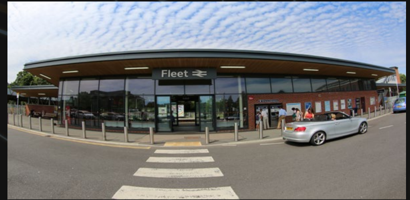
Fleet Mainline Railway Station
