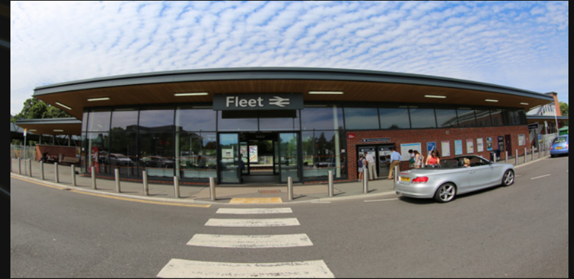
Fleet Mainline Railway Station
