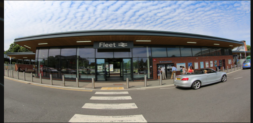
Fleet Mainline Railway Station
